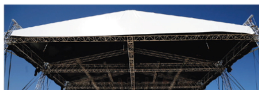
ROOF TRUSS SYSTEM 15x8 Mtr
